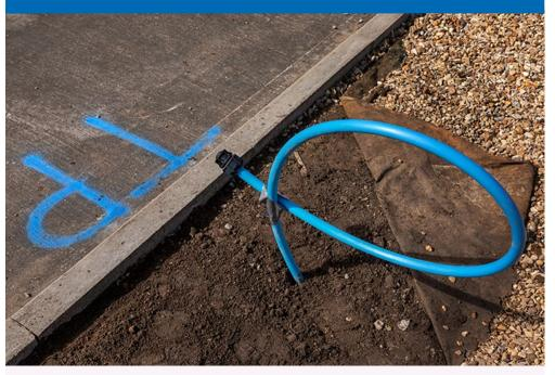
A minimum 2 metres of pipework exposed and the end of your tailpipe sealed with a compression cap coming up from ground level on the edge of your boundary and/ or at the agreed connection point. This will be marked by us with a blue 'TP'. We will endeavour to be at least 2 metres clear from any street furniture i.e. lamppost, telegraph pole, etc.
