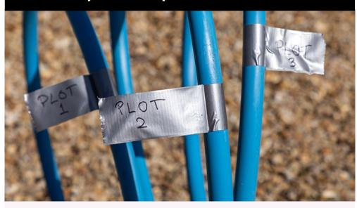
**Pipework is individually labelled if there are multiple connections,** to show which property or plot each pipe will supply (plot numbers are fine).
