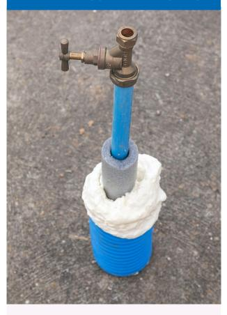
A correctly installed and approved internal stop-tap is in place (see pages 11, 12 & 13).
