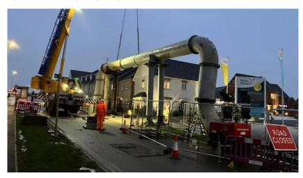
Figure 16: Temporary overland pipe as part of rising main repair
