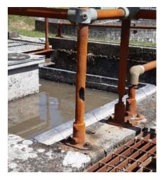
In recent years we have identified a root cause of failure in our sewer networks as hydrogen sulphide attack of concrete sewers. This occurs at the discharge point of rising mains, where the anaerobic conditions within the rising main mean that hydrogen sulphide is released, reacting with water in the sewers to create sulphuric acid which corrodes both concrete and steel.
