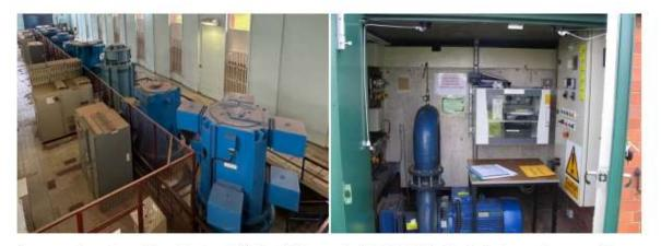
Images above show Hampton Loade's high lift pump hall at 12 MW of installed pumping capacity, and a small distribution booster of 30 kW capacity. Both of these sites would be treated equally in the booster stations per length of main variable, counting as one site each, which is clearly not reflective of the power costs nor the capital maintenance requirements.
