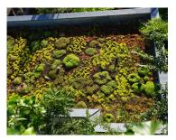
Green roofs or walls enable surface water to filter through the vegetation.
