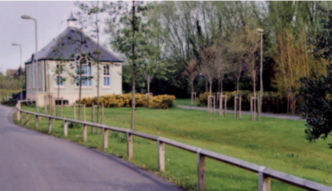
Witney, Oxford – Filter strip and swale
