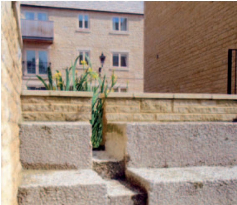
Riverside Court Stamford – outfall to River Welland
