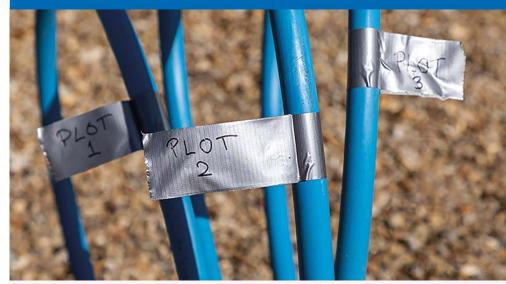
Pipework must be individually labelled if there are multiple connections, to show which property or plot each pipe will supply (plot numbers are fine).
