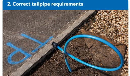
A minimum 2 metres of pipework exposed and the end of your tailpipe sealed with a compression cap coming up from ground level on the edge of your boundary and/ or at the agreed connection point. This will be marked by us with a blue 'TP'. We will endeavour to be at least 2 metres clear from any street furniture i.e. lamppost, telegraph pole, etc.
