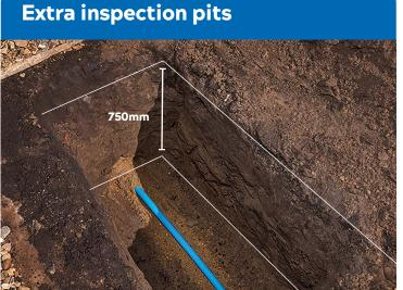
**A minimum of one inspection pit at the point of entry into the property** with the pipework exposed, showing the insulation and ducting. Extra inspection pits are required to every 10 metres when the distance from point of entry to your boundary is over 10 metres (or a half way inspection pit when the total distance is between 11m-19m). Use the drawing on page 3 for reference. *Please note the insulation must be a minimum 9mm thickness*.
