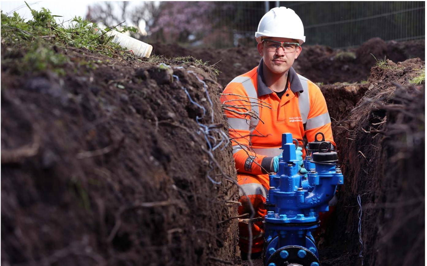
Where possible, water mains will be constructed with a minimum cover of 750mm from the top/ crown of the main or 900mm in verge or unmade ground. When in a footpath or footway, the centre of the main should be 690mm from the kerb face (as per [NJUG guidelines](#)).
