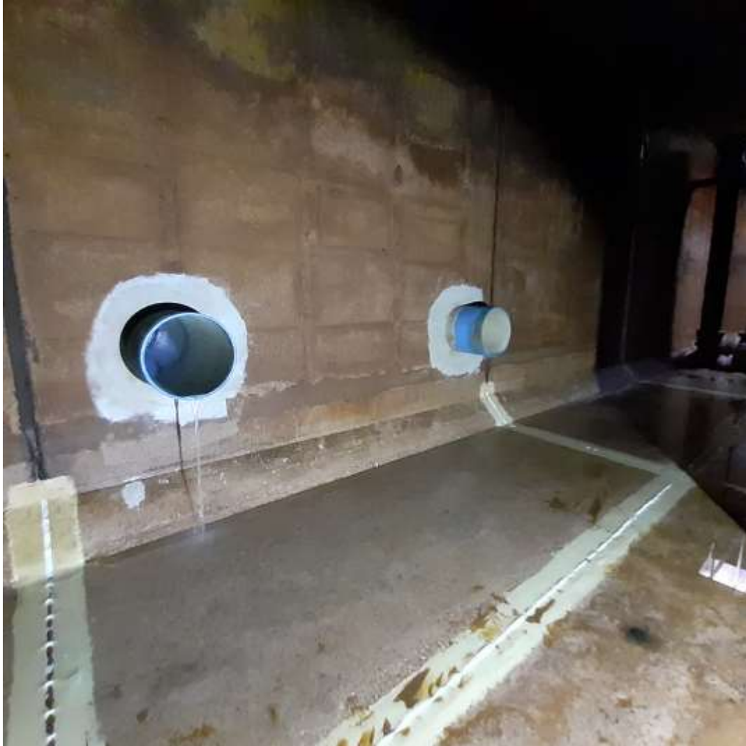
New outlet pipes
