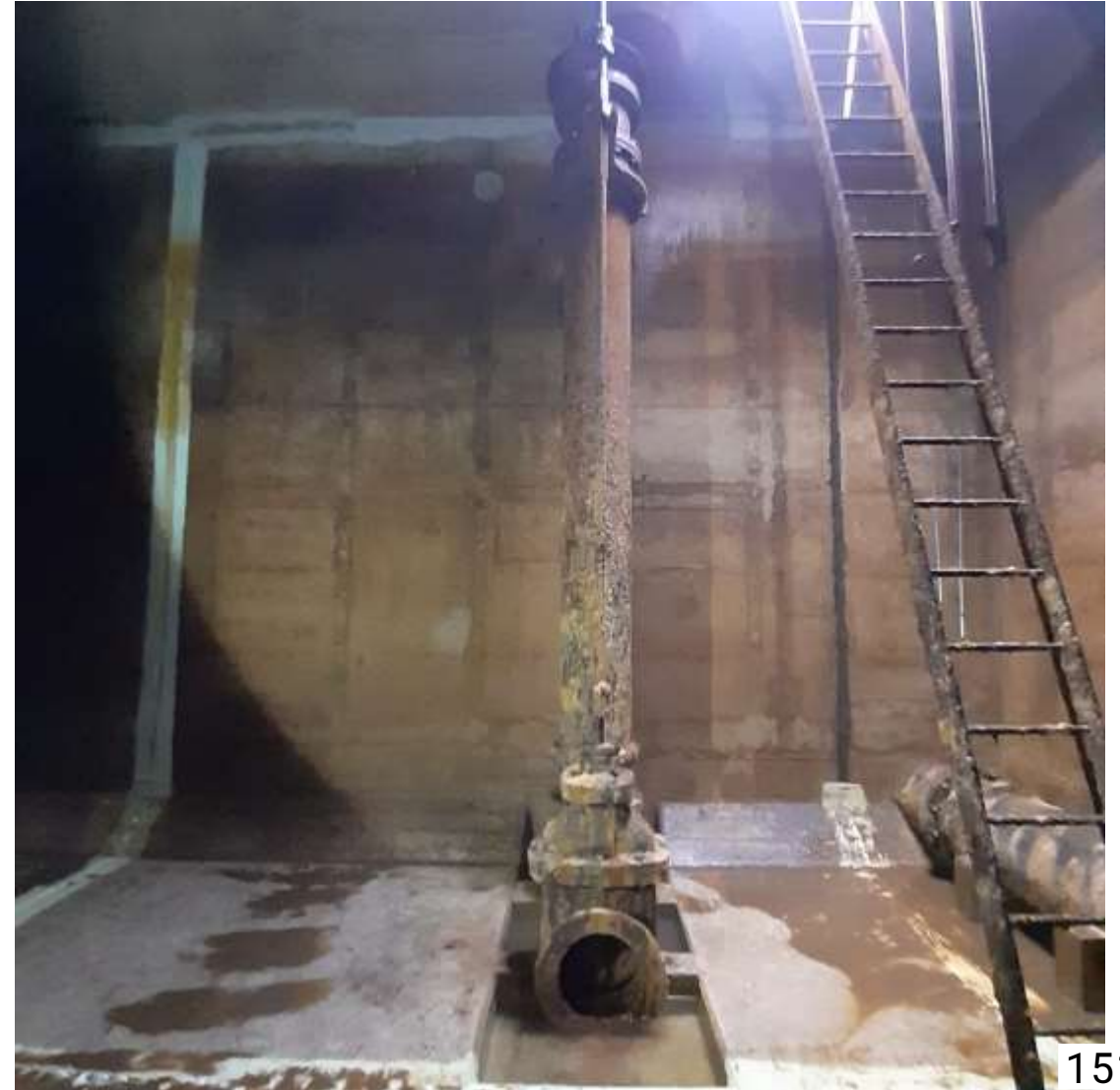
Washout and overflow pipework
