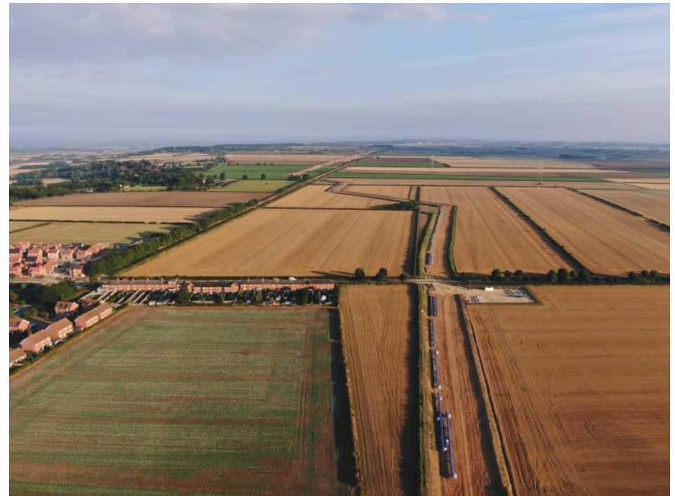
Figure 74 Construction of our strategic pipeline
