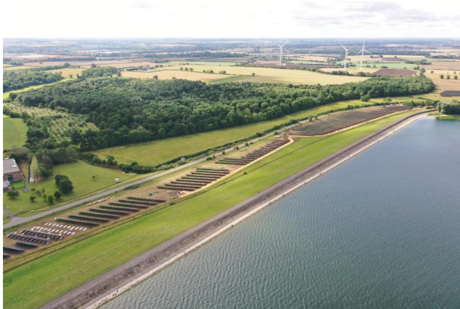
Figure 75 A solar array at one of our reservoirs
