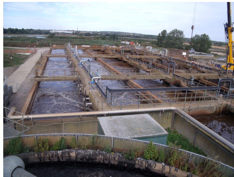
Figure 1 Bedford WRC aeration settlement lanes
