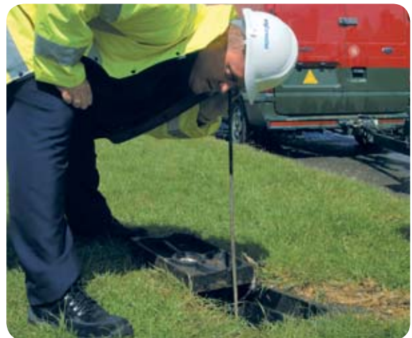
↑ Listening for leaks in a water main
