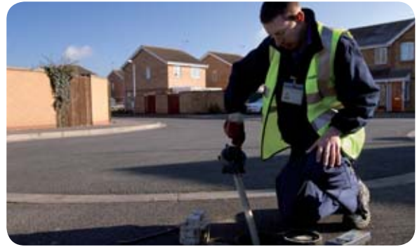
↑ A water meter being fitted
