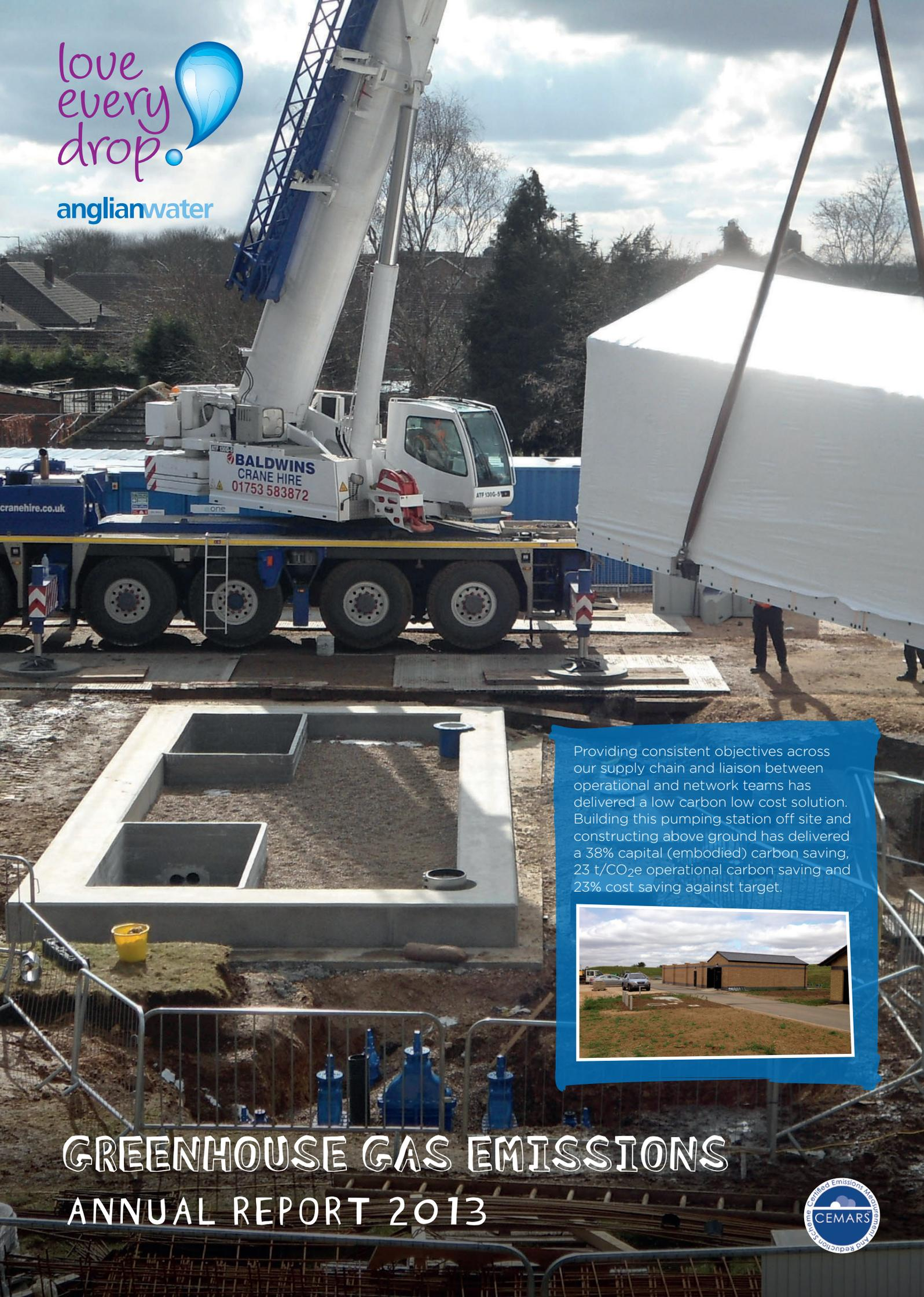
Providing consistent objectives across our supply chain and liaison between operational and network teams has delivered a low carbon low cost solution. Building this pumping station off site and constructing above ground has delivered a 38% capital (embodied) carbon saving, 23 t/CO<sub>2</sub>e operational carbon saving and 23% cost saving against target.
