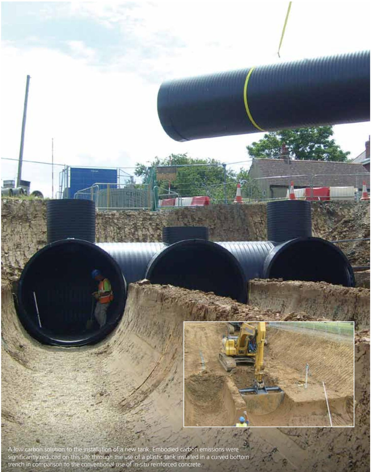
A low carbon solution to the installation of a new tank. Embodied carbon emissions were significantly reduced on this site through the use of a plastic tank installed in a curved bottom trench in comparison to the conventional use of in-situ reinforced concrete.
