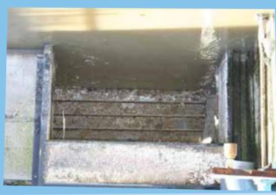
The incoming used water is made up of 99% water and 1% solids. It's important to remove the solid material as soon as possible to prevent blockages and damage to the machinery.
