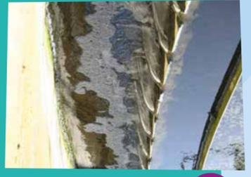
The sewage then flows into large round, funnel shaped tanks where the primary settlement takes place. Soil and poo sinks to the bottom of the tank because it's heavier before being piped away from the bottom.
