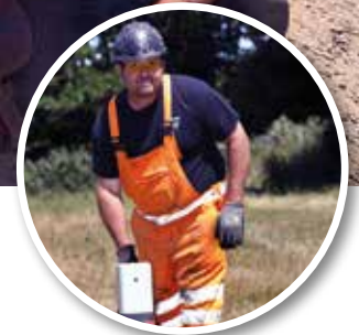
Jansen Broddle tracking the directional drill head.
