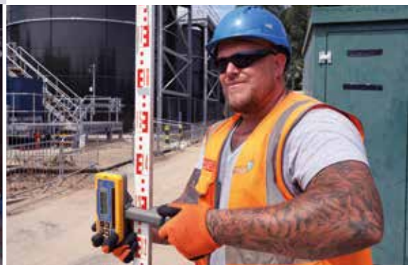
R G Carter (Civils) Foreman Dean Lamb checking finished concrete levels.
