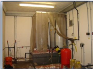
Build off site dosing system with integral chemical tank and bund.
